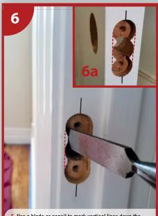
6. Use a blade or pencil to mark vertical lines down the sides of the 3x overlapping Ø 24-25mm holes on door and
