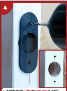
4. Insert the plastic Strikebox/drilling template into the edgebore hole and use as a guide to drill 2x Ø 3mm pilot holes above and below edgebore hole.
