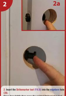
Close door tightly then press the pointed Strikemarker tool into the jamb to mark a mounting position for the strikeplate.
