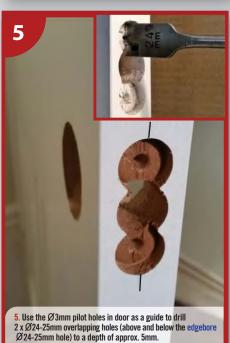
2 x Ø24-25mm overlapping holes (above and below the edgebore Ø24-25mm hole) to a depth of approx. 5mm.
